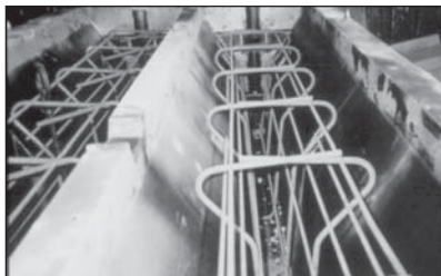
WWR used in highway median barriers.
