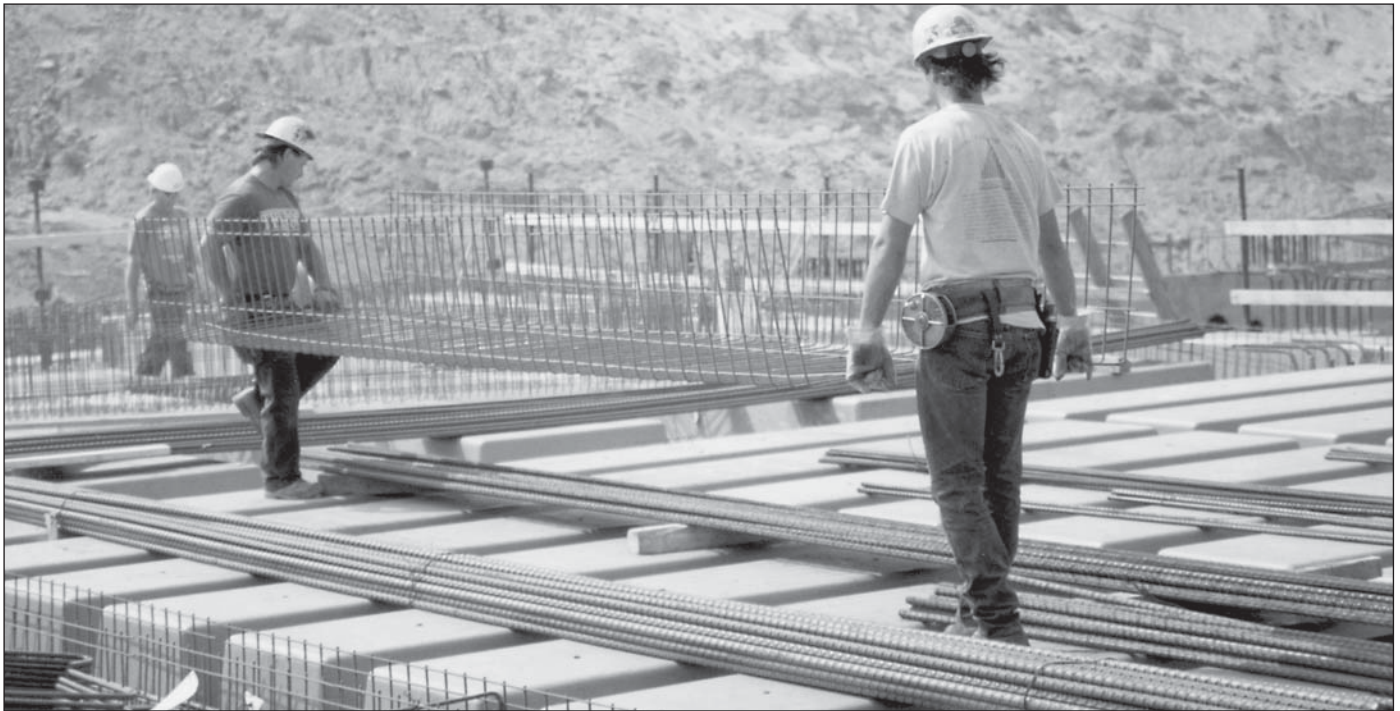
Placing a shear cage of welded wire reinforcement in a concrete girder for a sports stadium.
