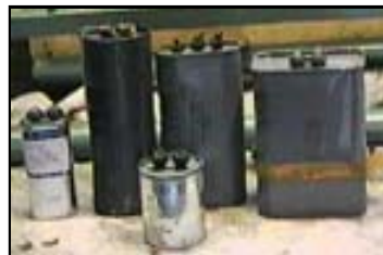
Typical Running Capacitors...GOOD! .....Starting cap...Bad!
